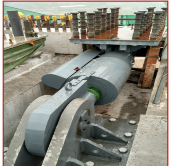
LUD 12000/300 Jinmeng Bridge (China)
