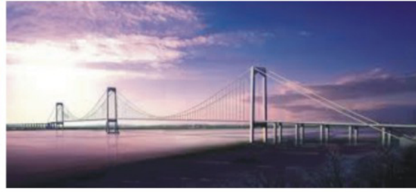
HIFLUID DEVICES FOR LANZHOU HEKOU YELLOW RIVER BRIDGE
