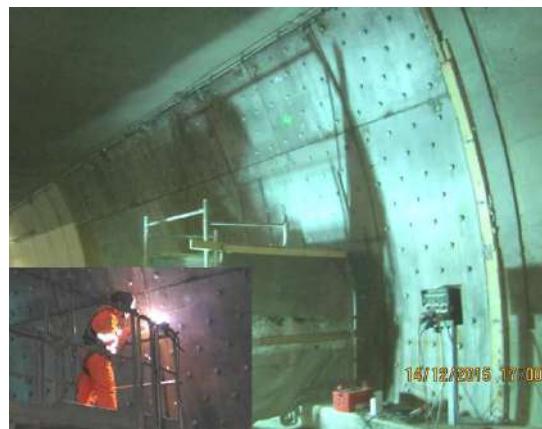
Figure 17. Reinforcement of sidewall by steel plates
