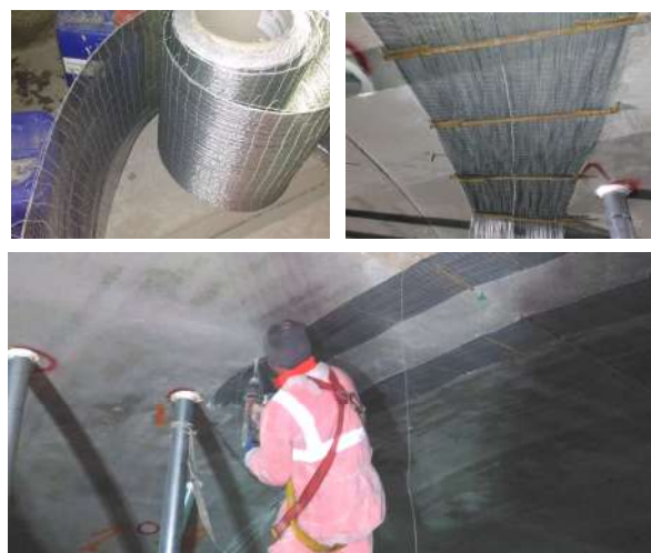
Figure 14. UHTSS steel net 200's application
