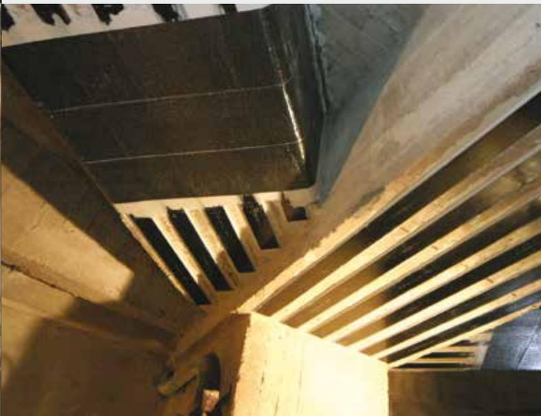
A photograph showing FRP sheets installed on a ceiling. The sheets are arranged in a grid pattern, with some overlapping. They have a light tan or yellowish color.
