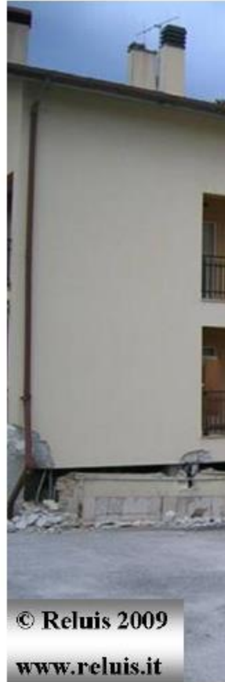
Soft storey mechanism
