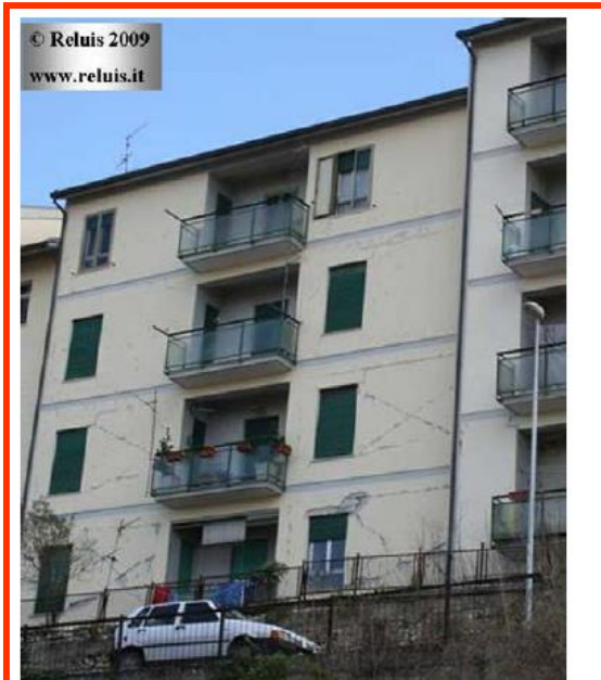
Infills damage: four stories R.C. building Evidence of typical diagonal cracks at the first two levels.
