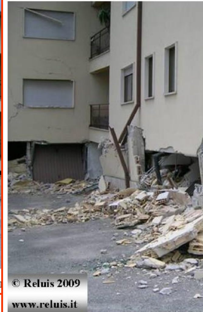
Soft storey mechanism
