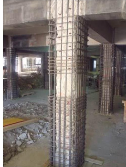
concrete casting to increase shear and flexural strength
