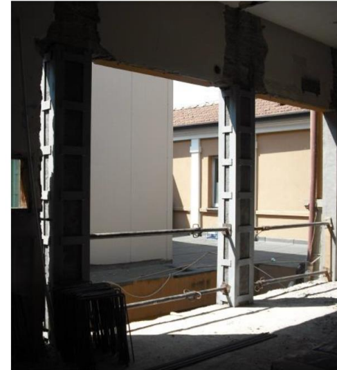
steel encasing for the same purpose
